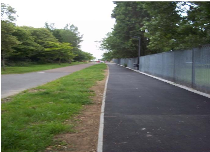
After: new pedestrian Way/ segregated cycle path created (Greendale cycle path
