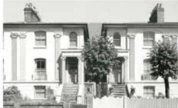
Listed buildings on Glengall Road
