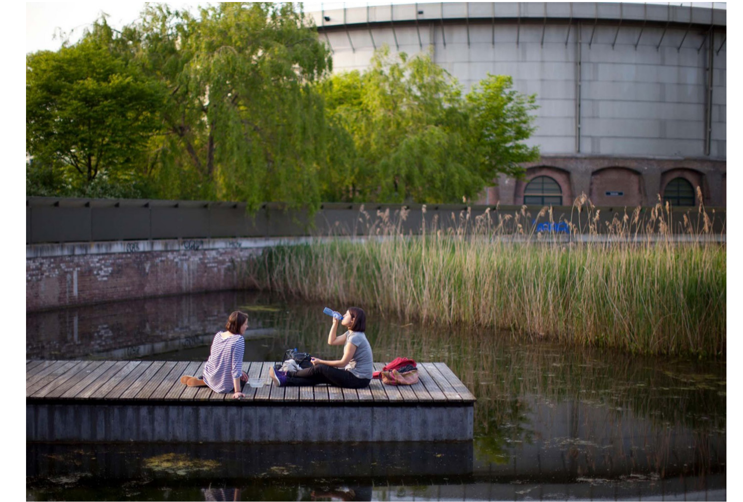
Gasholder converted to natural pool, Amsterdam
