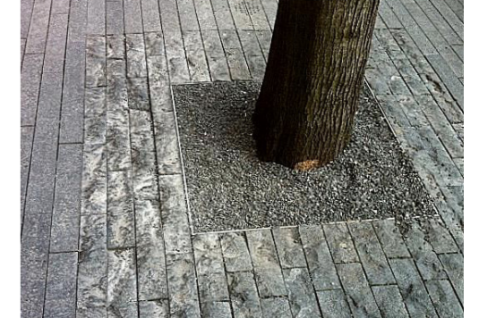
Recessed and integrated tree pit
