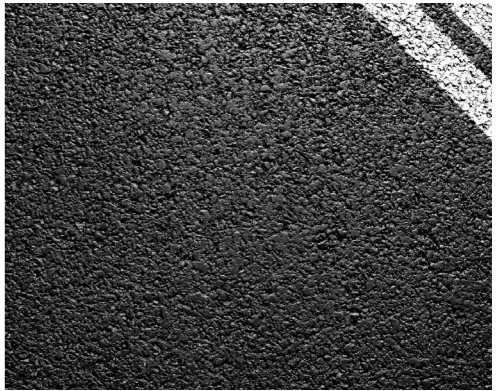
Asphalt to highways
