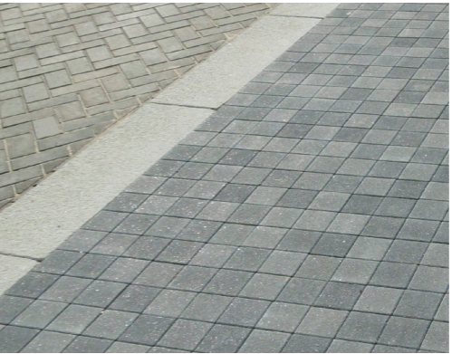
Flush granite kerbs and block/brick paving to roads and service areas
