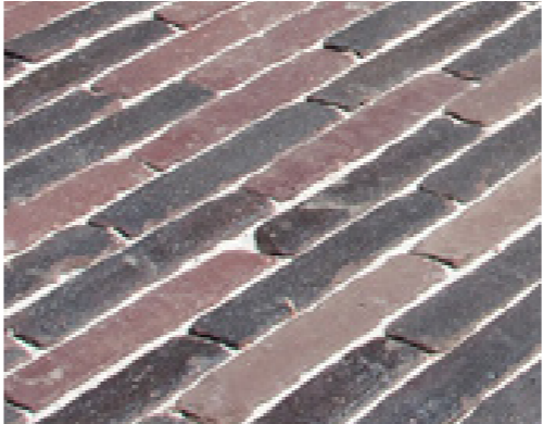
Brick paving to spill-out areas
