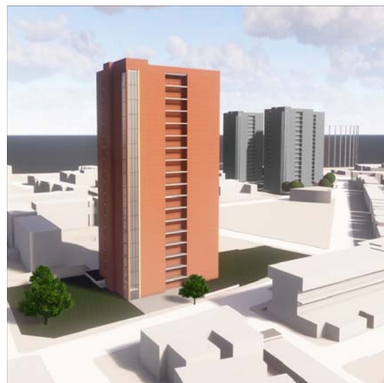
Aerial view from Junction between Ledbury Street and Commercial Way
