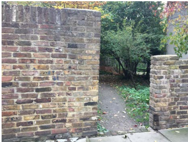
SOLID WALL ALONG BROCKHAM ROAD BOUNDARY
