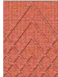
Hall block feature wall with detail brick pattern inspired by the roof forms
