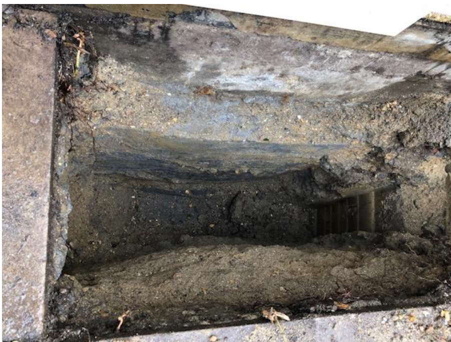
Underpinning to the rear of 81 Manor Grove
