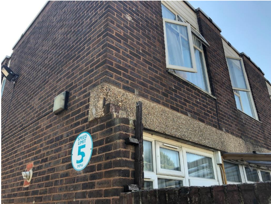
Photograph 13 – Projecting brickwork wall at supports to first floor rear beams.
