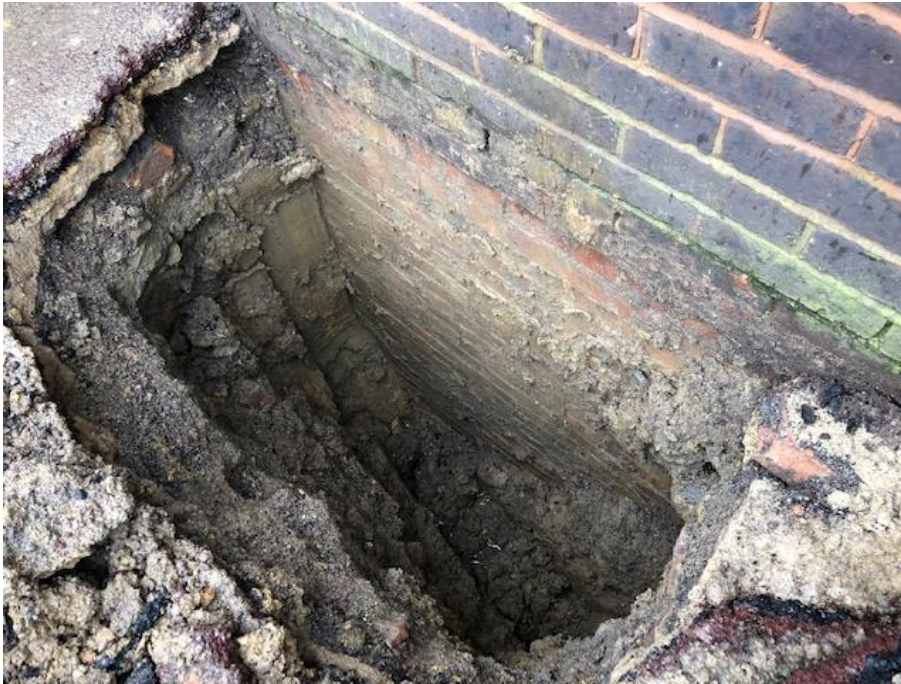
Deep foundations to the flank wall of 81 Manor Grove.
