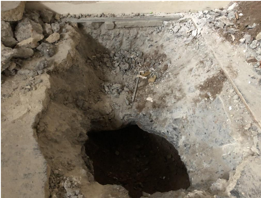
Internal trial pit carried out at 81 Manor Grove
