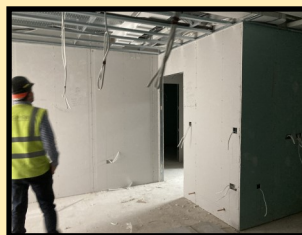
Plasterboard to walls
