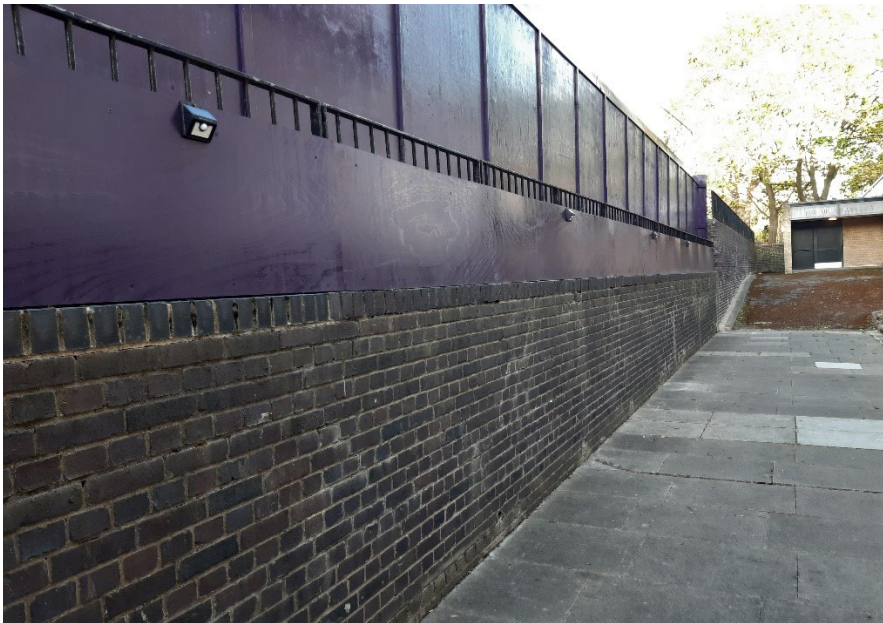
Additional lighting to hoarding
