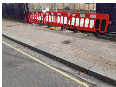
Internal concrete cross over to allow access and egress
