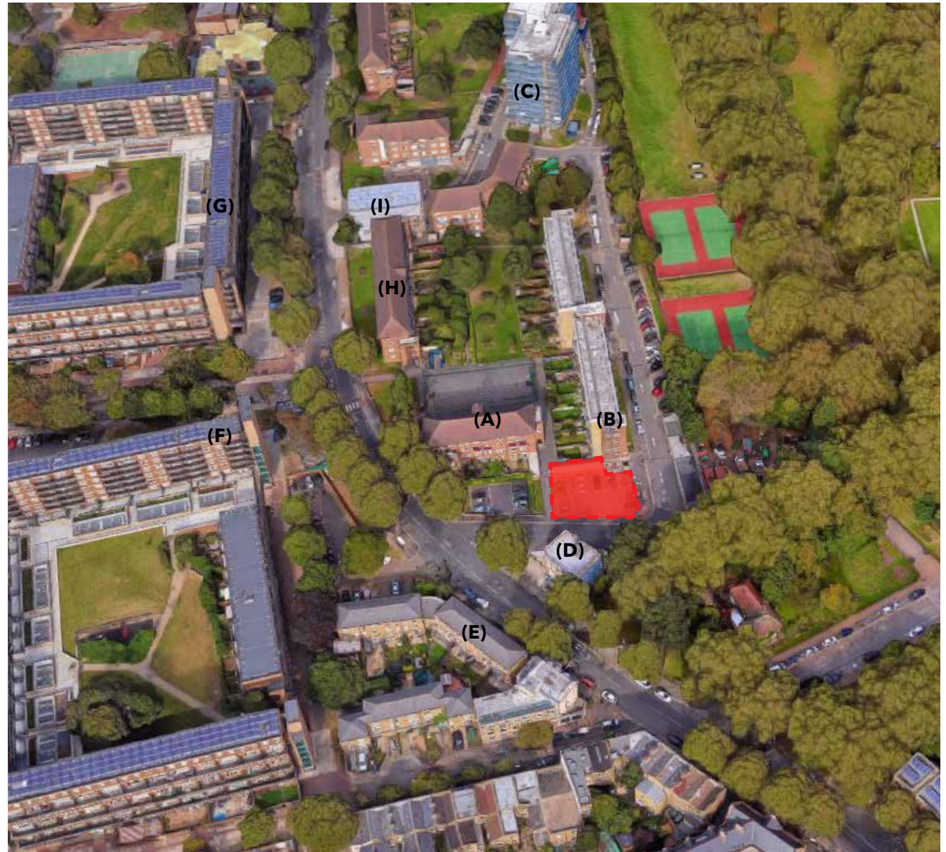
Aerial view with storey heights
