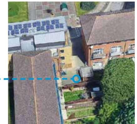
4) Between Glebe House and Cornick House
