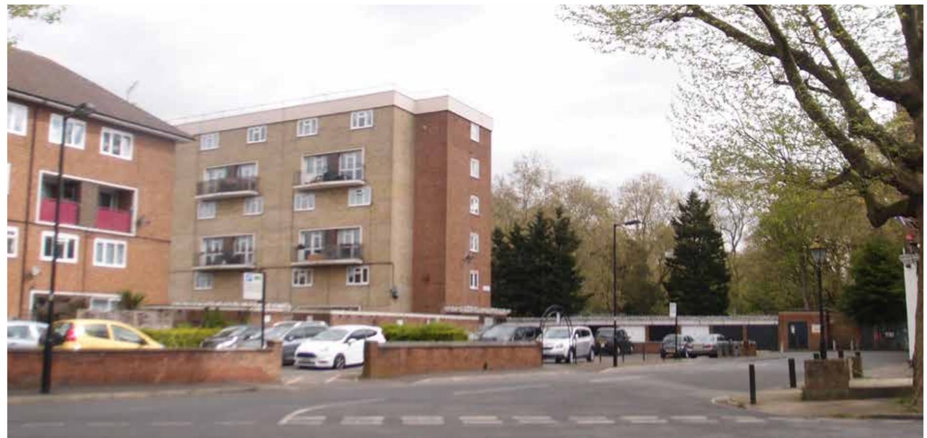
The site from Southwark Park Road - from above and from the road - looking towards Stalham Street.
