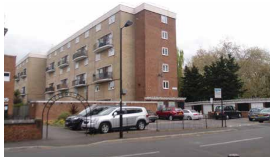
1. View from Stalham Street - southwest corner of the site.
