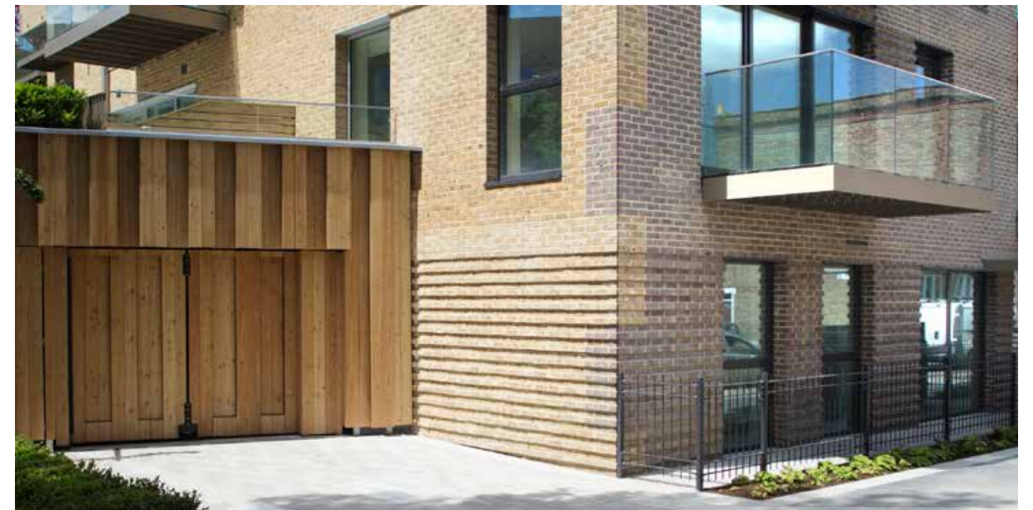
Podium Parking - Trafalgar Place, Southwark, London
