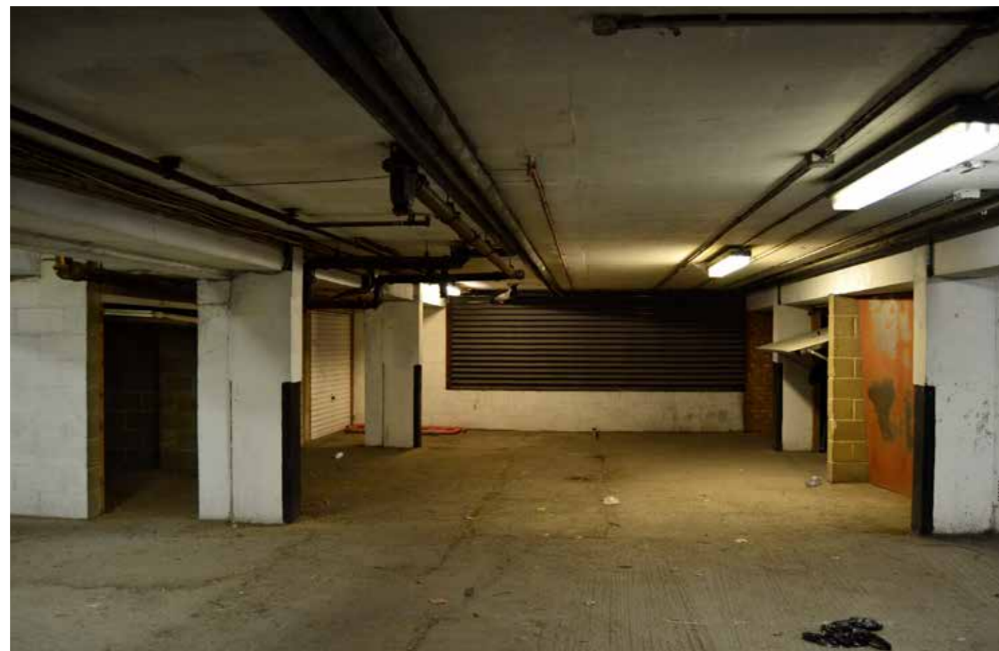
2) Internal view of existing garages looking north
