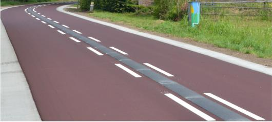
This type of separation deters vehicles from driving in the cycle lane while maintaining access to driveways. This can also be used as a guiding marking at an intersection.
