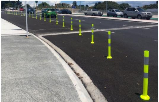
This type of treatment can be used instead of permanent kerb build-outs on a temporary basis.
