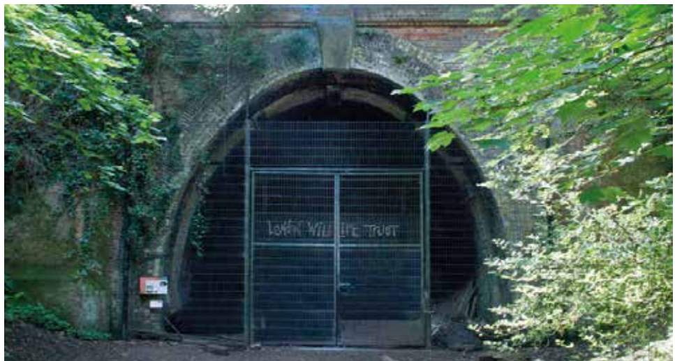
Railway tunnel, photograph by Sara Moiola
