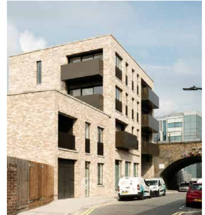
Light buff brick with metal projecting balconies. Karakusevic and Carson. Great Eastern Buildings.
