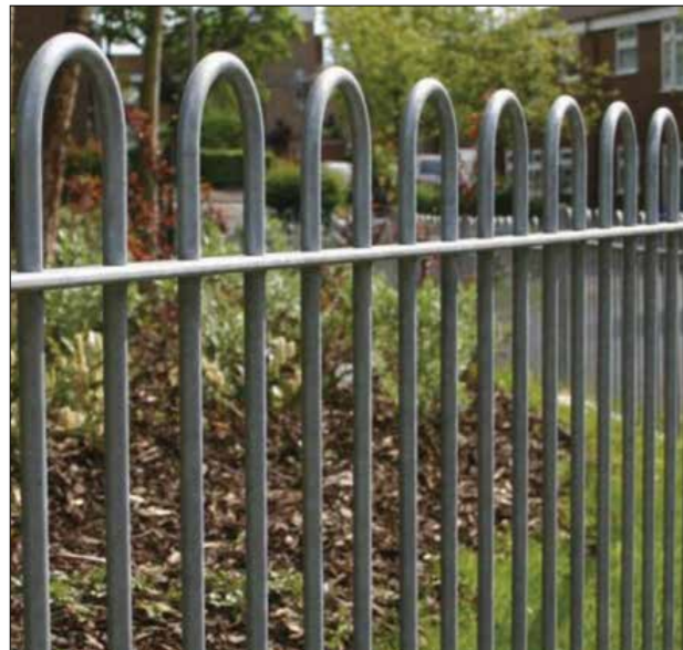
Bow Top Metal fencing to play area
