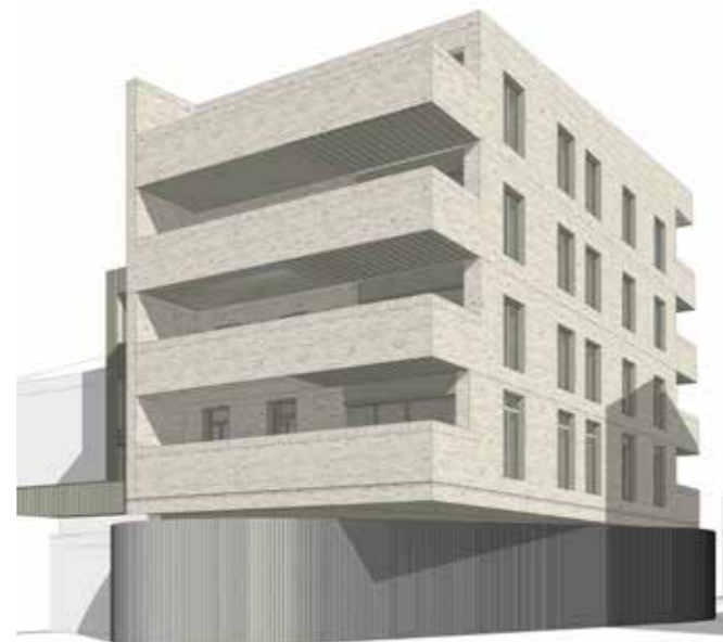
Balcony along the whole facade
