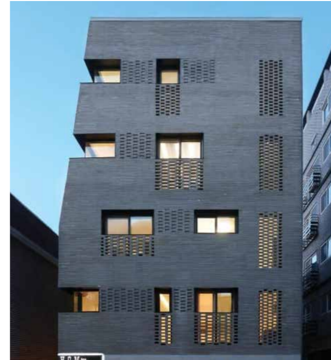
Slanted facade, corner recessed balconies with high parapet.
