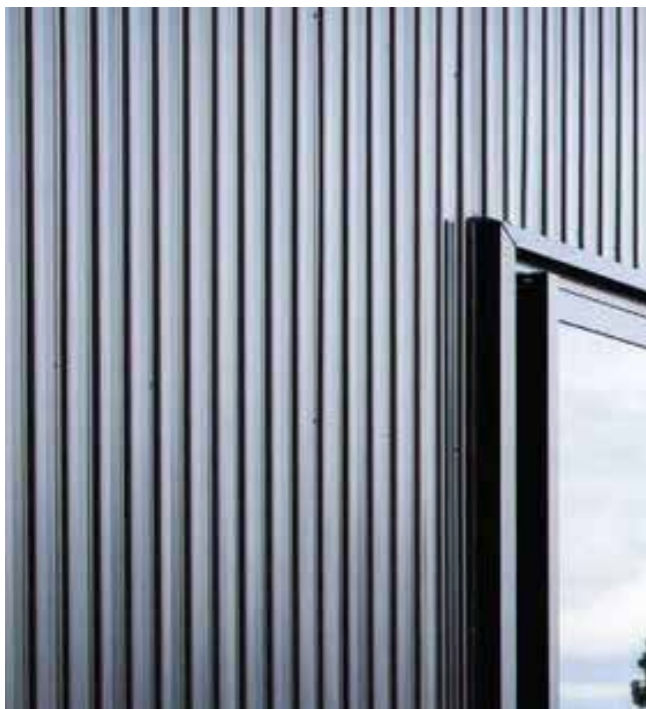
Warm grey undulated metal sheet. Clear difference between both building uses, Tenants' Hall and residential.
