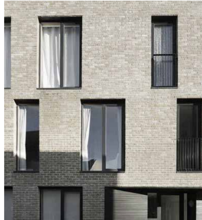
Full height windows with dark frames and reveals
