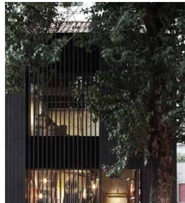
Opening protected by lattice during evenings
