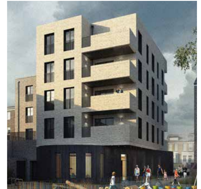
West elevation in lighter brick with darker mortar
