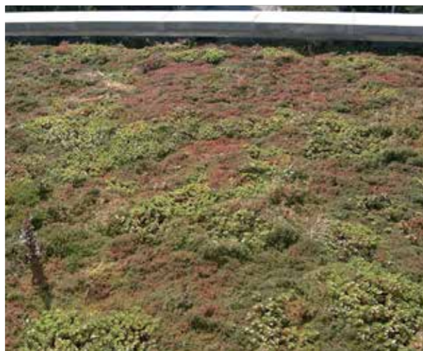
Extensive green roof - sedum mat and wildflower plugs
