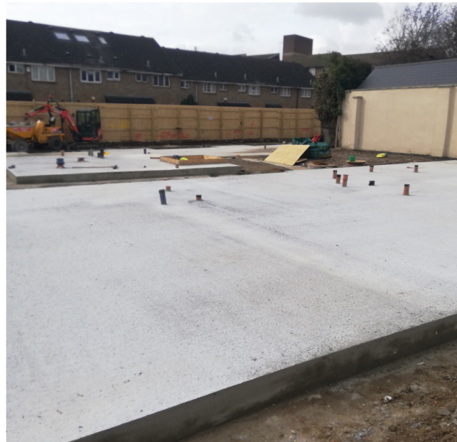
Installation of foundations
