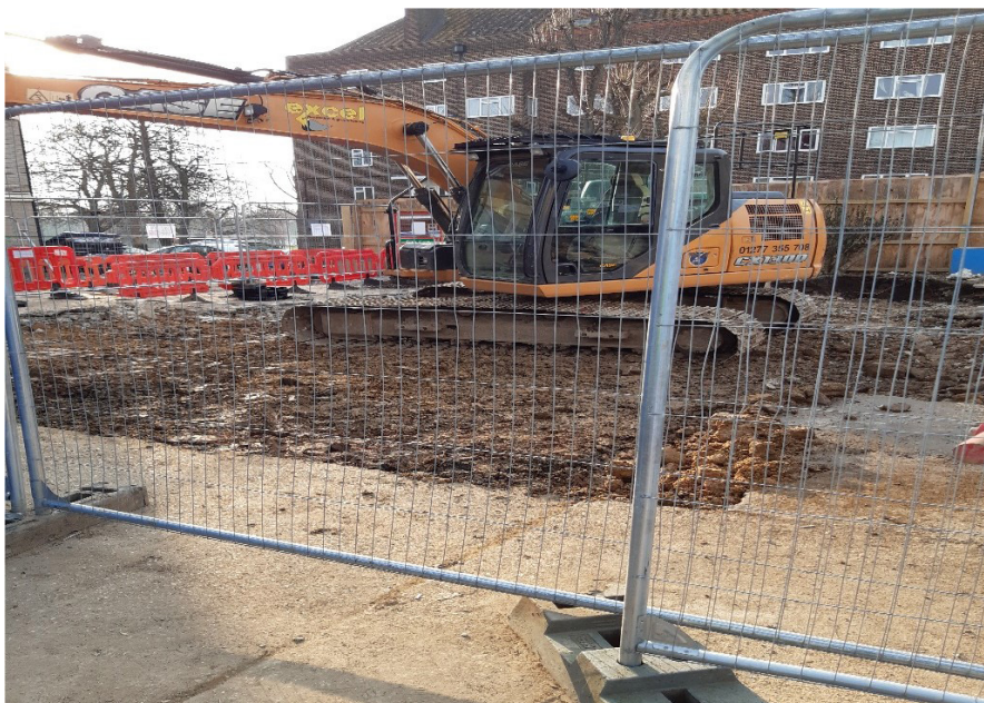
Reduce dig and slab adjacent Rye Hill Park
