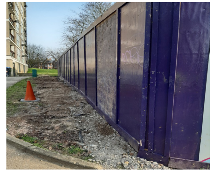
Hoarding alteration - north elevation
