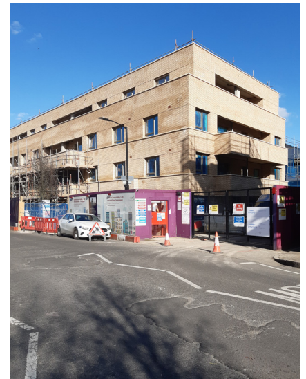
Scaffold removal - West elevation
