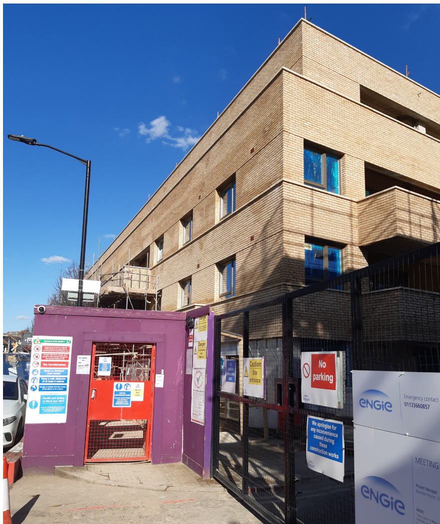
Scaffold removal - West elevation
