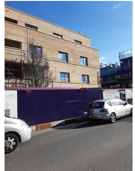
Scaffold removal - Northwest elevation
