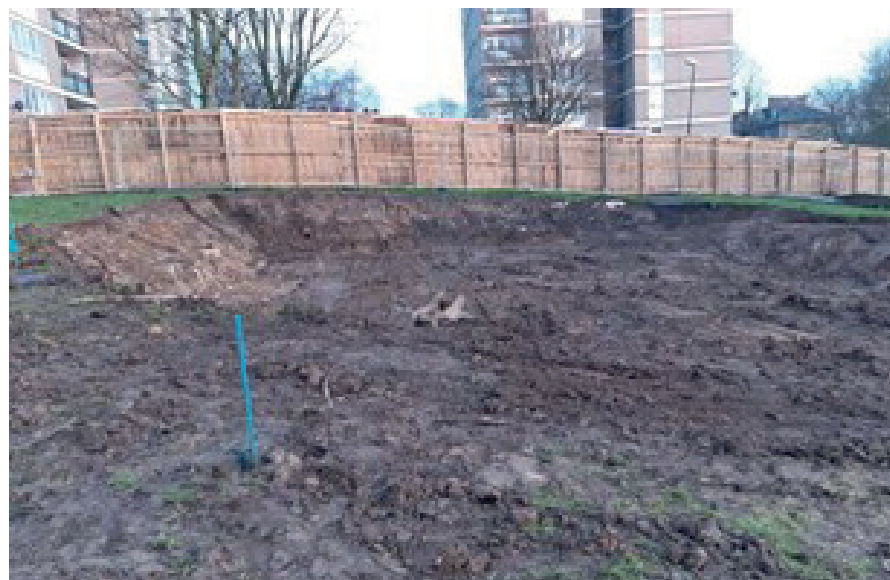
Reduce dig across site
