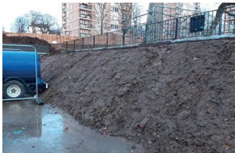
Garages removal and battering
