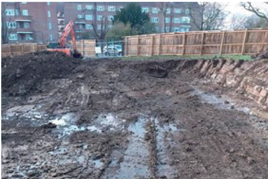
Reduce dig at Block A
