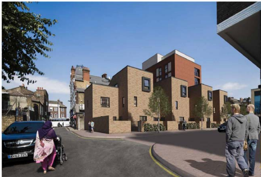
OKR 8: 16/AP/4589 UNDER CONSTRUCTION
