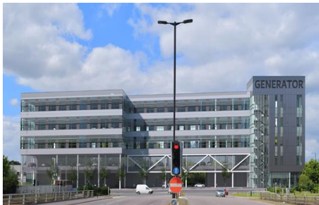
The Generator, Park Royal – St George PC expect 2021
