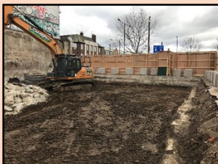
Site ready to lay the recycled piling mat.
