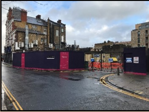
Site Entrance and hoarding—Kinglake Street
