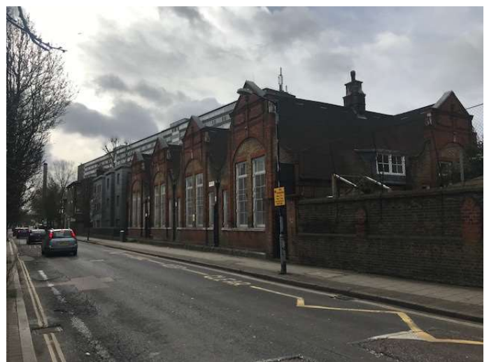
Figure 22 Former Boys School, Flint Street (now English Martyrs Primary School)
