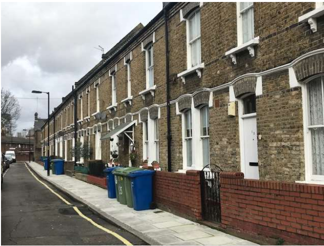
Figure 25 The addition of unsympathetic porches and boundary treatments
