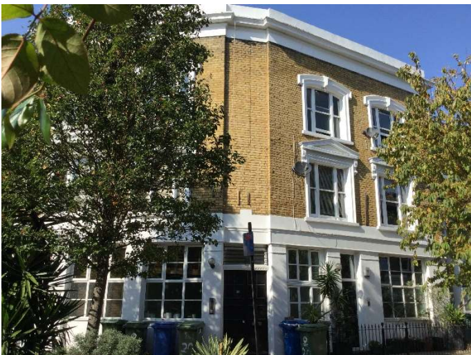
Figure 21 The Globe former public house, Darwin Street
