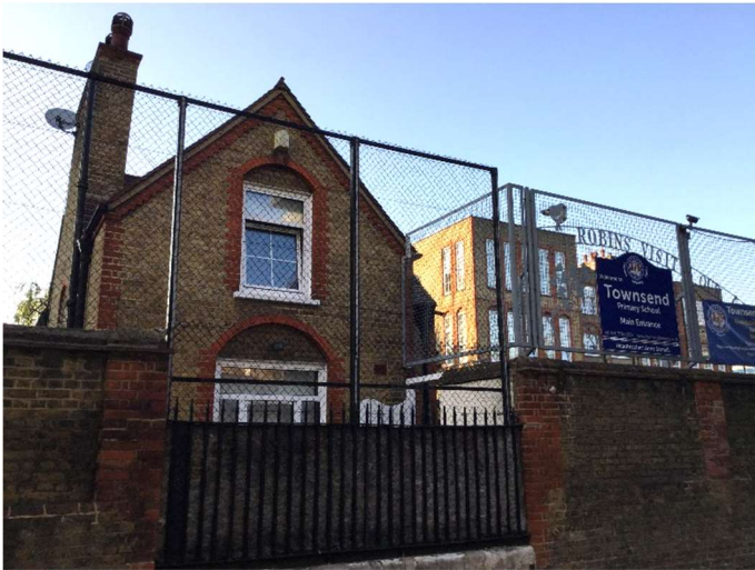
Figure 16 Former school keepers house and Townsend Primary School, Townsend Street
