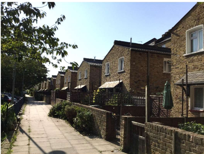
Figure 24 Rear elevations of outriggers of Nos 3a–53b Darwin Street, with entrances to flats onto Mason Street
