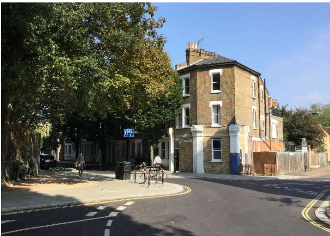
Figure 42 No. 83 Balfour Street, with chamfered edged former shopfront that meets the junction
