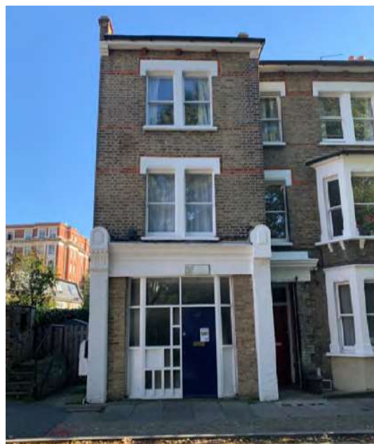
Figure 41 No. 67 Balfour Street with former shopfront
