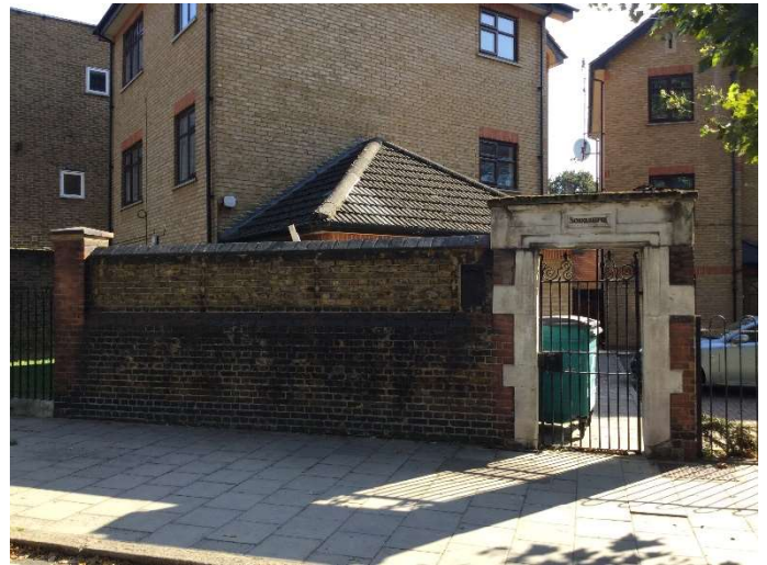
Figure 32 Entrance to the Schoolkeepers cottage (demolished) in the extant former Paragon school wall
