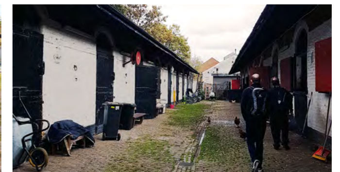
Existing stables building
