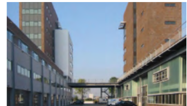
Business Center Kaap Nord, Amsterdam, The Netherlands, 2005
