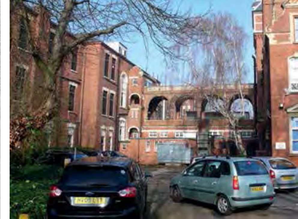
Contemporary use of grounds: parking and plant
