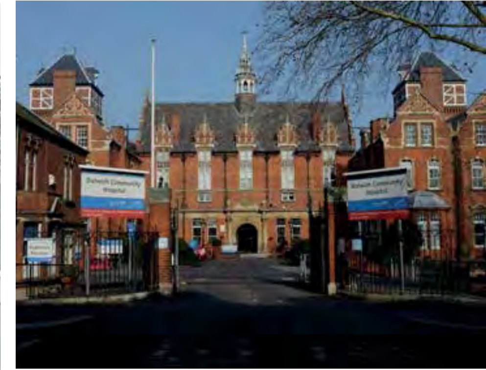
Current view to the main entrance to Dulwich Community Hospital
