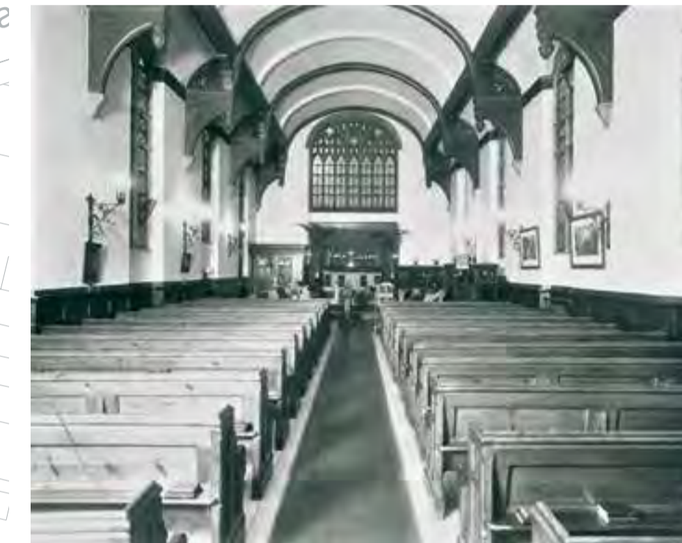
Original chapel with 28ft high barrel vaulted ceiling and ornamental wooden principals
