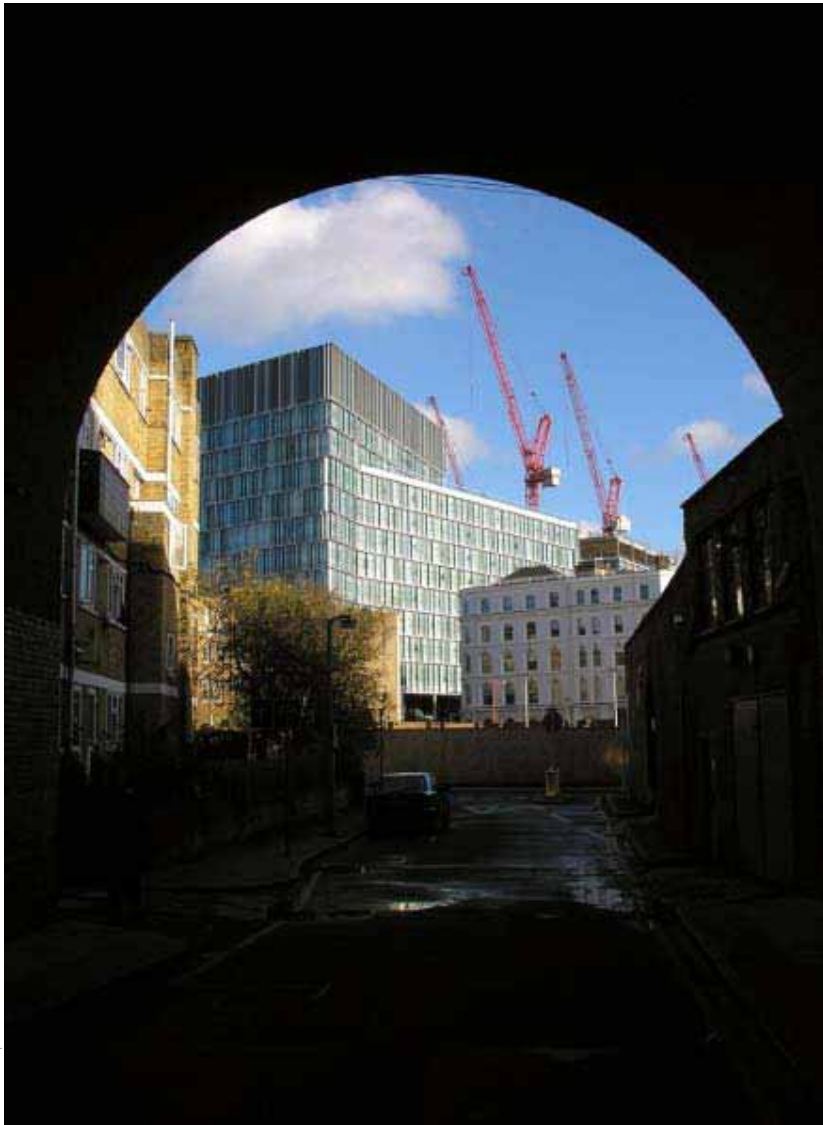
Blue Fin Building seen through Viaduct Arch
