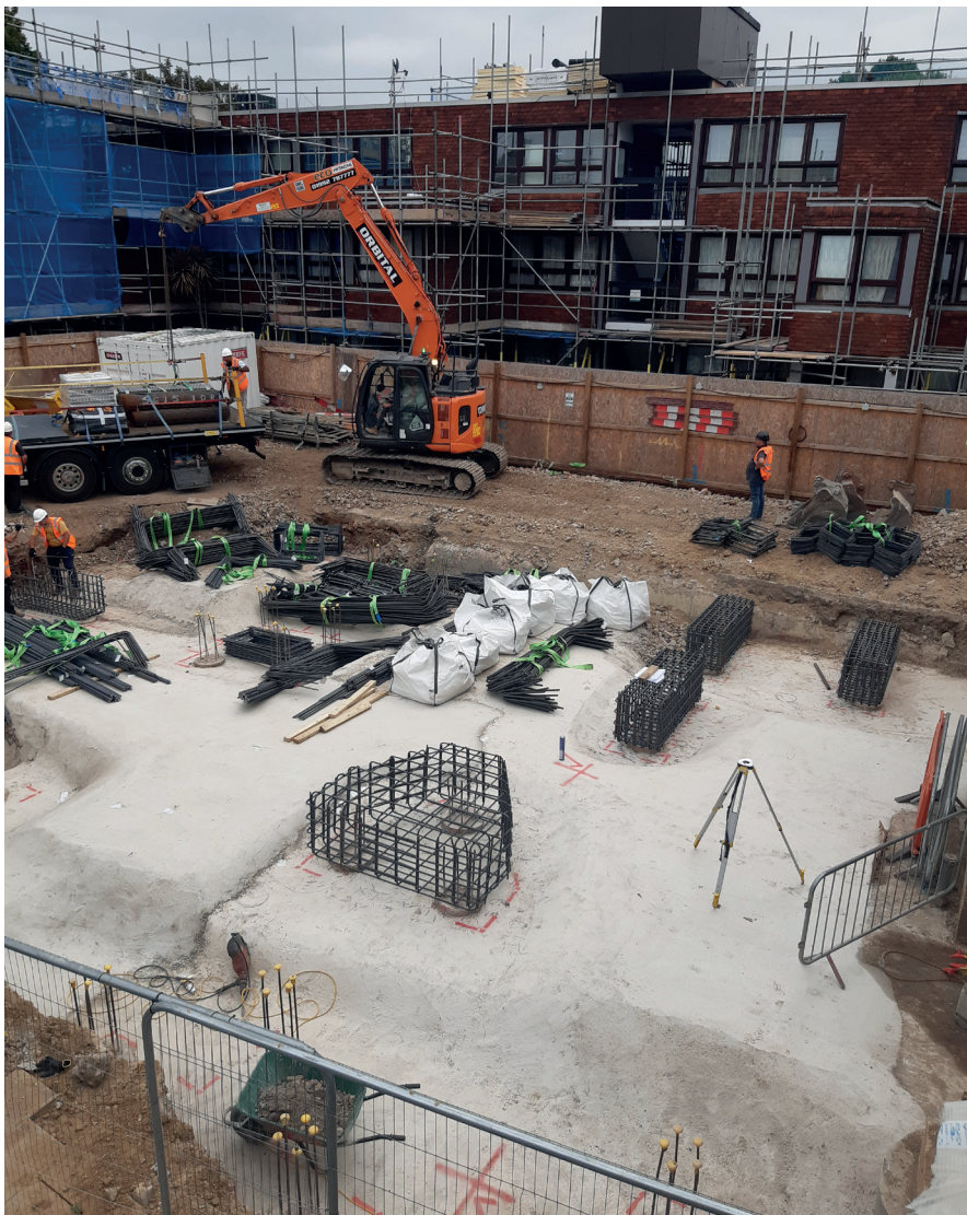
New community centre piling - Phase 2
