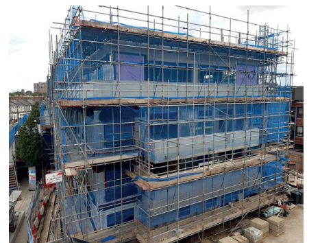
External view of our progress
