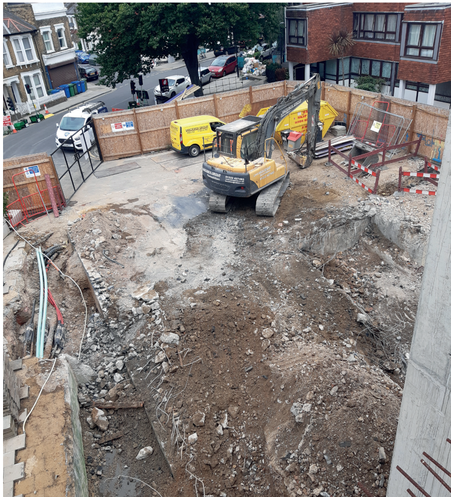
Demolition of the existing substation is now complete
