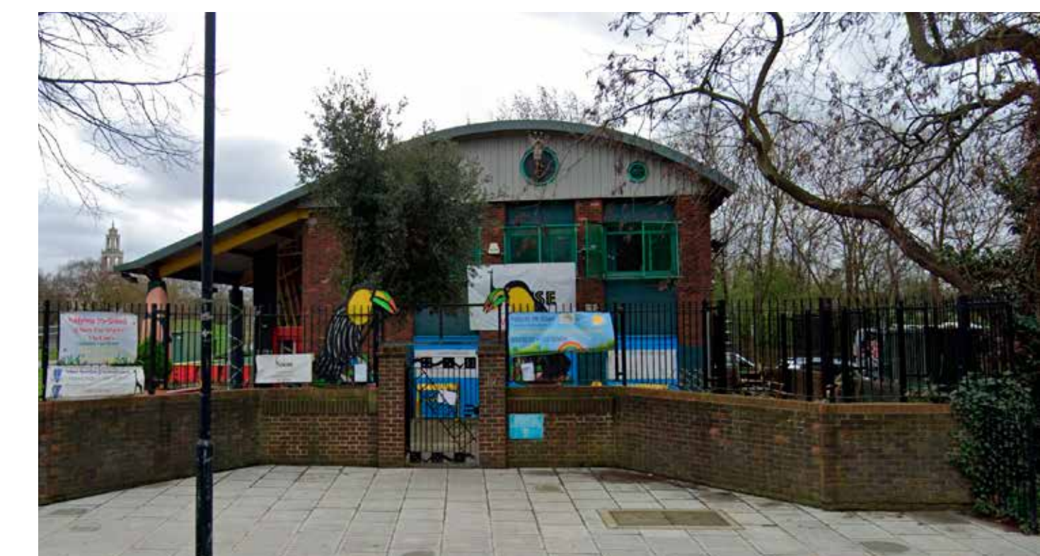
EXISTING BUILDING TO BE REMOVED IN PHASE 2 (DATE TBC)
