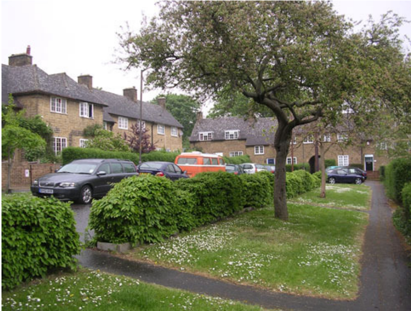
Cul-de-sac (9-45 Casino Avenue)
