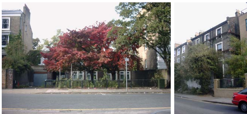
Figure 41 Vacancy and dereliction in De Crespigny Park: 13-15, left, and 28, right
