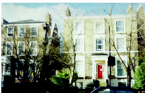
Figure 34 De Crespigny Park: part of a once more extensive estate of large villas each in its own spacious grounds
