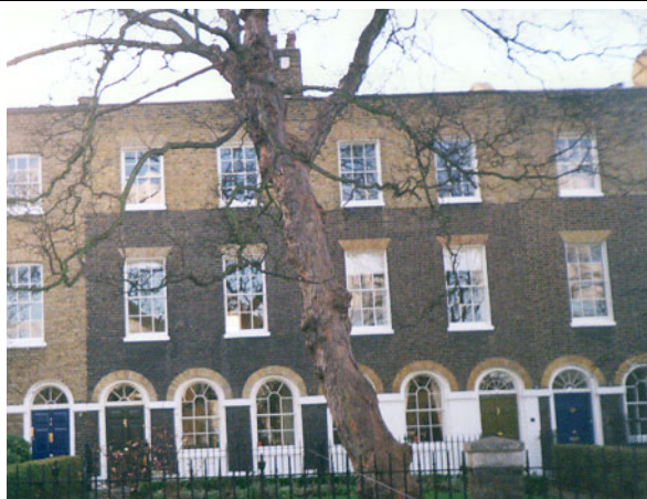
Figure 17 18-60 Grove Lane; a late 18 th century terrace. Front garden planting and railings are integral to the quality of the group.
