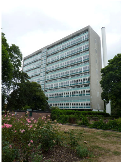
Lakanal Tower, part of the Sceaux Gardens Estate, forms a contrast with the terraced bungalows close by
