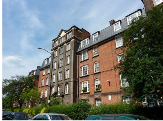
The proportions employed in the Peabody buildings respond well to the scale of the Green itself
