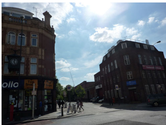
The Athenaeum is a key corner building in need of refurbishment
