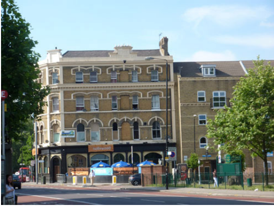
The Nollywood, formerly the Redstar, is a local landmark, facing down the length of the central green space
