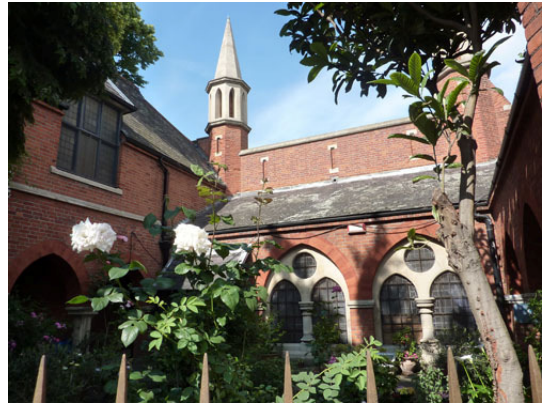
St. Mary's Greek Orthodox Church, Camberwell New Road: an important marker building
