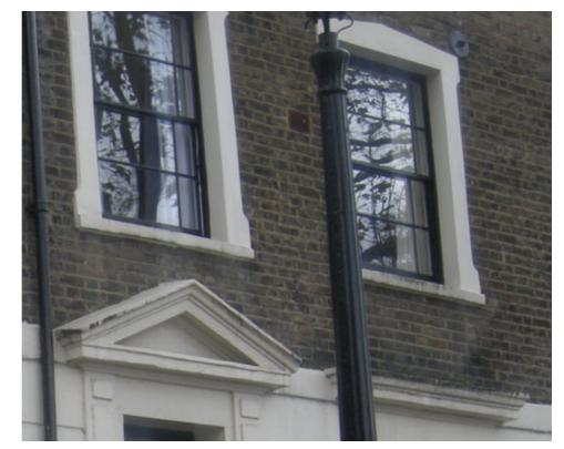
Figure 14 Erosion of stucco mouldings in Merrick Square
