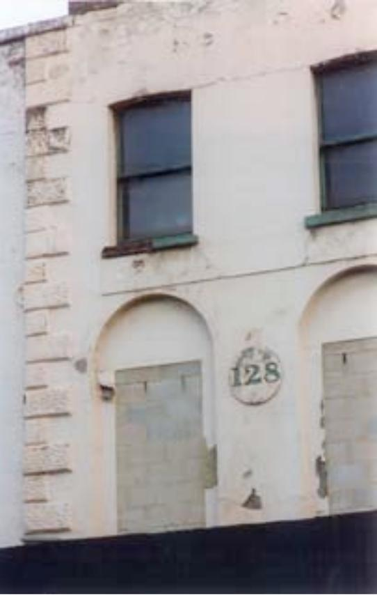
Figure 14 Stucco detailing to No 128 London Road
