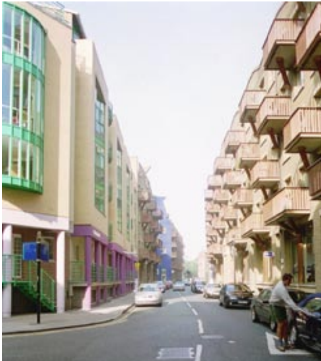
Figure 10 Many new developments are based on devices used in former wharf buildings. Queen Elizabeth Street looking west from Shad Thames.
