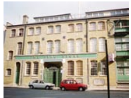
Figure 30 21-29 Queen Elizabeth Street: buildings at Jubilee Yard maintain most of their warehouse features.
