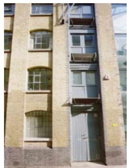
Figure 9 The regular disposition of openings is a distinguishing feature of the warehouse aesthetic. The "Coriander" Building,, No. 20 Gainsford Street.
