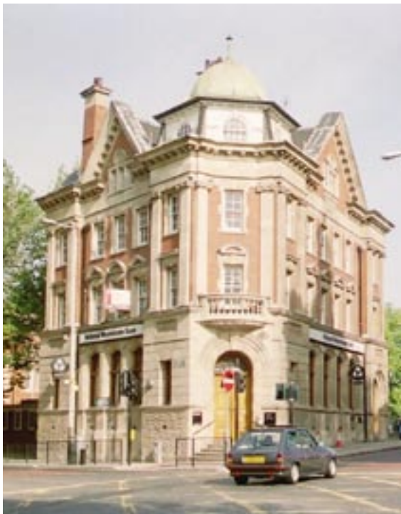
Figure 11 Buildings on Tooley Street have an elaborate civic style characteristic of the late 19th century. The former London & Counties Bank, 185 Tooley Street.
