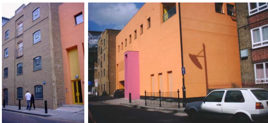
Figure 17 (left) 1950s/60s concrete framed buildings refaced, at 77 Bermondsey Street in "traditional" style, and
