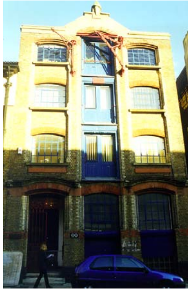
Figure 10 Warehouse building, 60 Weston Street, showing the typical narrow elevation, divided into tall bays with a prominent central loading bay, gables and hoists.
