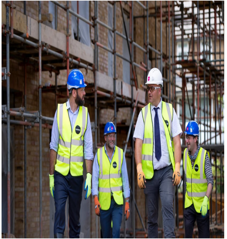
Block A The Townhouses – Just leaving Block A through what Will become the rear gardens. Following a successful tour of site Each house now the staircases are installed and internal walls are under construction.
