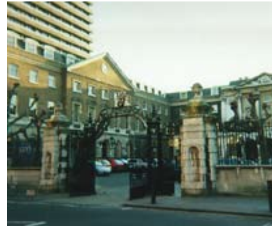
Figure 37 Forecourt of Guy's Hospital: the prospect to the entrance and flanking wings of the original hospital is very fine, but car parking is intrusive.
