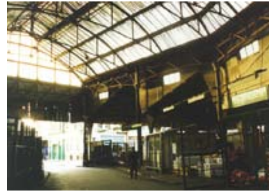
Figure 32 Interior of Borough Market – an internal street environment.
