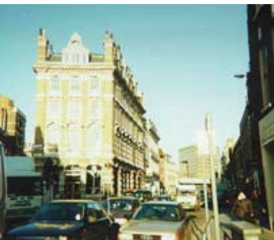
Figure 16 Looking towards Town Hall Chambers: once the site of St. Margaret's Church, the historic market place, and now the setting for the Southwark War Memorial.
