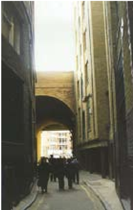
Figure 29 The canyon-like quality of the eastern end of Clink Street as it passes below the railway into Bankside.
