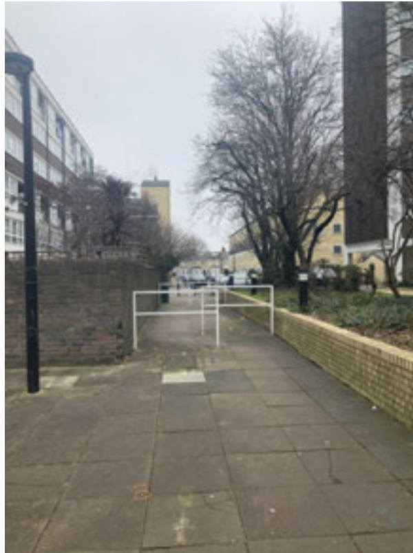
Plate 59: Looking South towards the Bells Gardens 2 Boiler House
