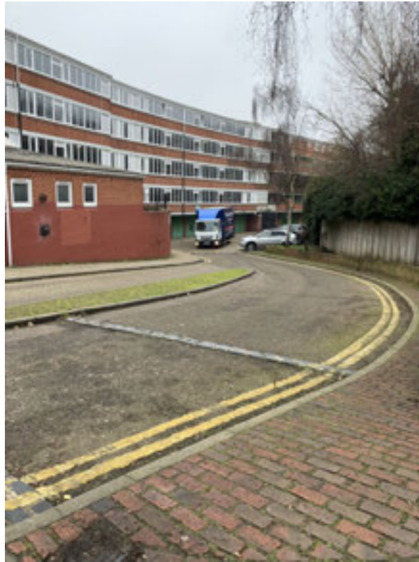
Plate 77: Changes in elevation in the area of the Boiler House
