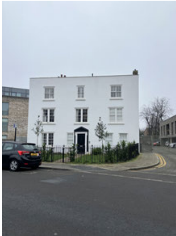
Plate 69: Early listed architecture at 4 Wood's Road
