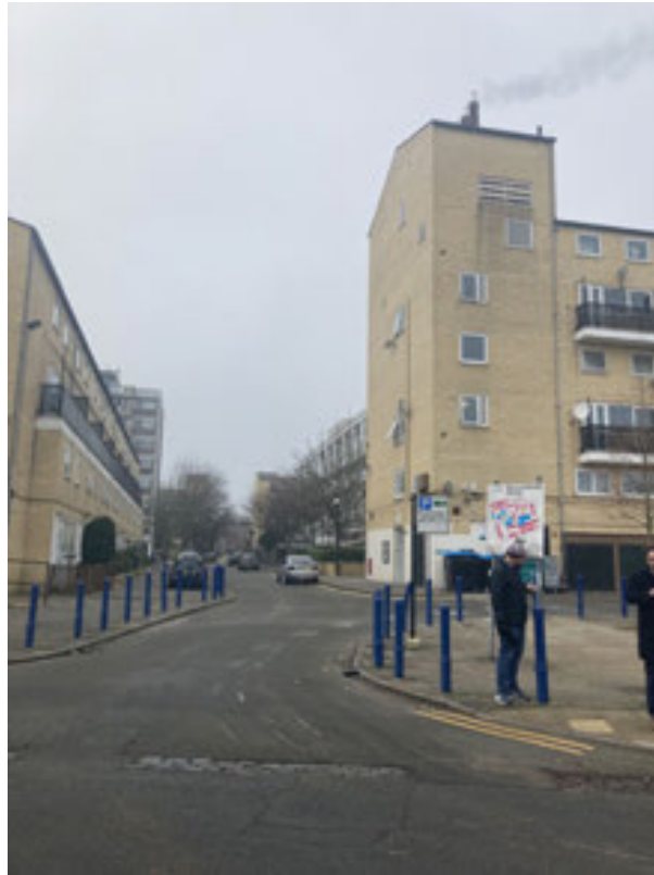
Plate 55: Entrance to the Boiler House for the DHN pipeworks at Bells Gardens Estate.
