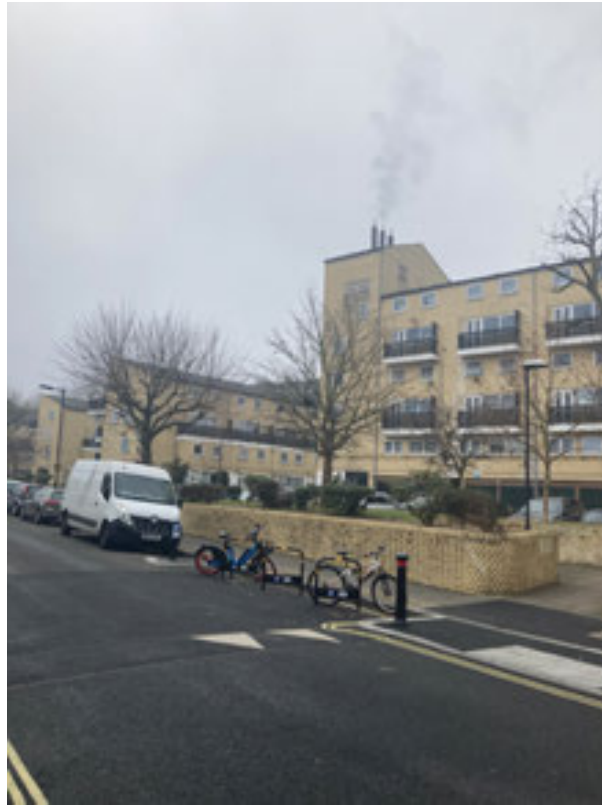
Plate 53: Route of DHN pipes south down Furley Road, to join the Boiler House at the Bells Gardens Estate
