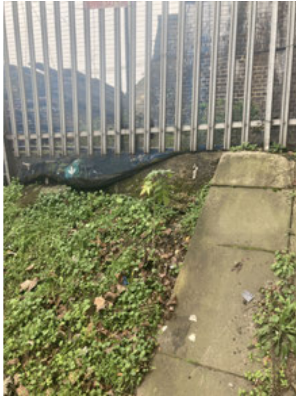
Plate 7: Elements of potential canalside architecture surviving by the Railway Bridge on Surrey Canal Road
