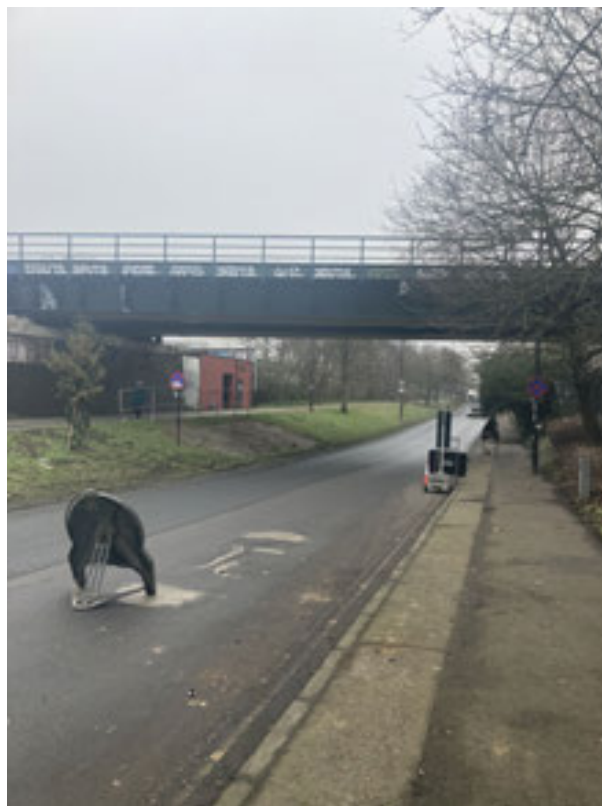
Plate 8: The westernmost railway bridge over Surrey Canal Road, the northern edge of the former canal can be seen in the raised bank to the left of the image.
