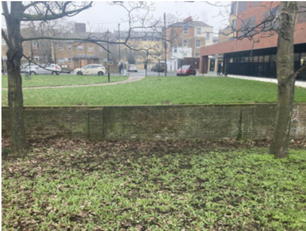
Plate 63: Looking East from Surrey Canal Walk to the change in height on Bonar Street at the historic location of Eagle Wharf beside the Grand Surrey Canal, The wall may be original architecture surviving from the canal.
