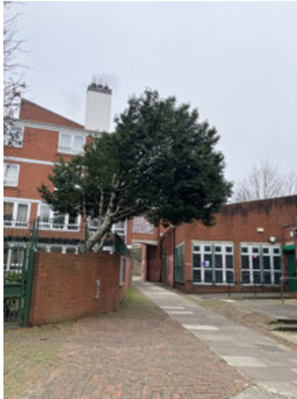
Plate 75: The DHN connection to the Boiler House on the Cossall Estate
