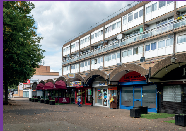
Existing shop fronts on Tustin Estate beneath Bowness House.
