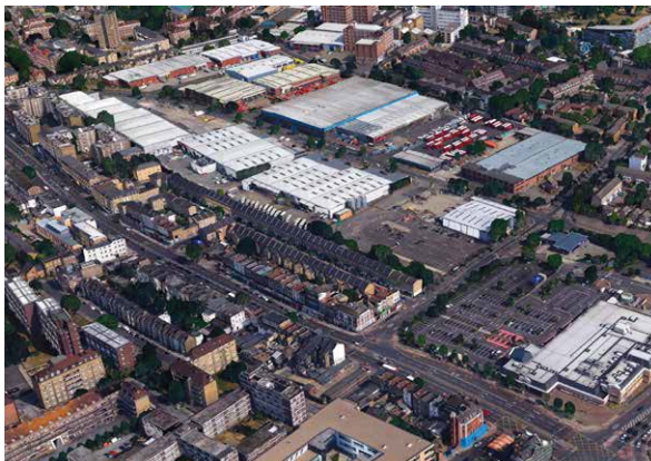
Mandela Way industrial area today (© Google)
