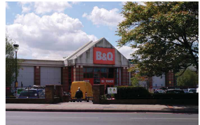
Cantium Retail Park
