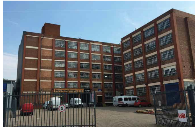
The Rich Estate work space cluster
