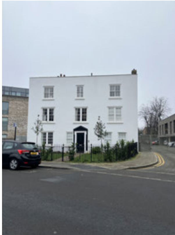
Plate 69: Early listed architecture at 4 Wood's Road
