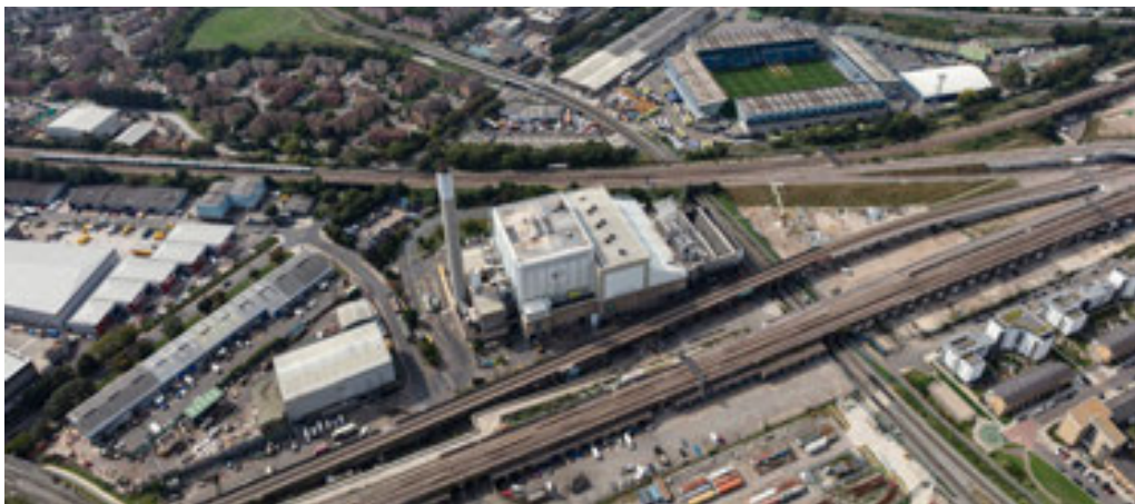
Figure 2. SELCHP facility where the main energy source is located
