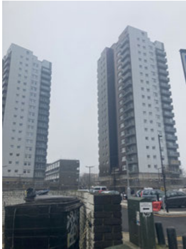
Plate 23: The Towers of the Tustin Estate on the east side of Ilderton Road
