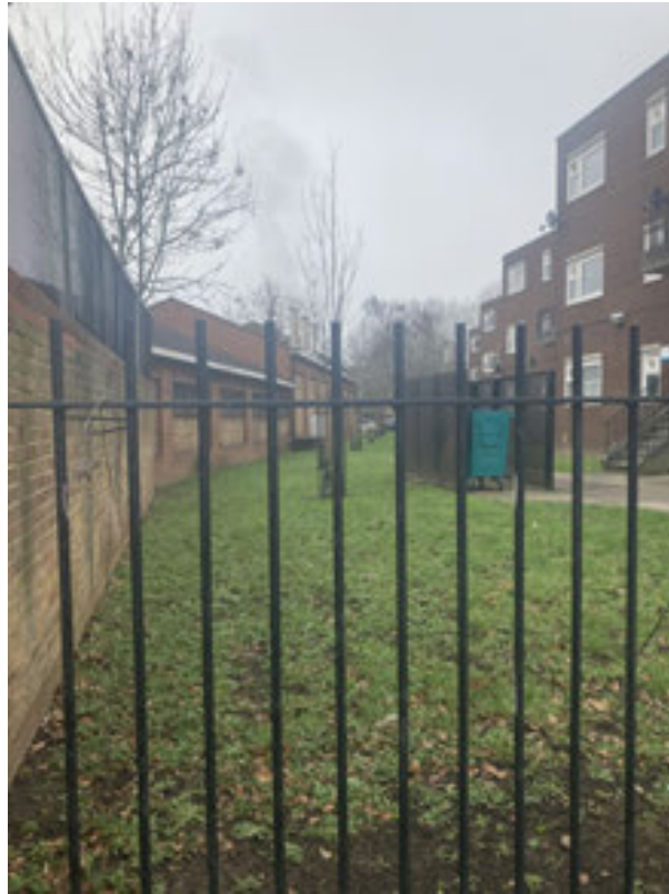
Plate 35: Route of the DHN, crossing Culmore Road and garden areas to the rear of Roman Way to connect with the Boiler House beyond
