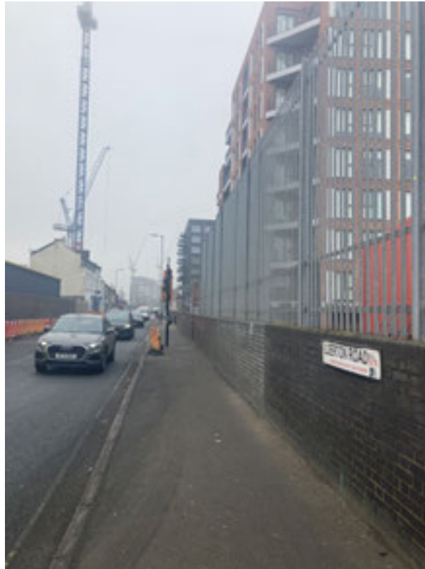
Plate 11: Looking South from the bridge at the junction of Surrey Canal Road and Ilderton Road
