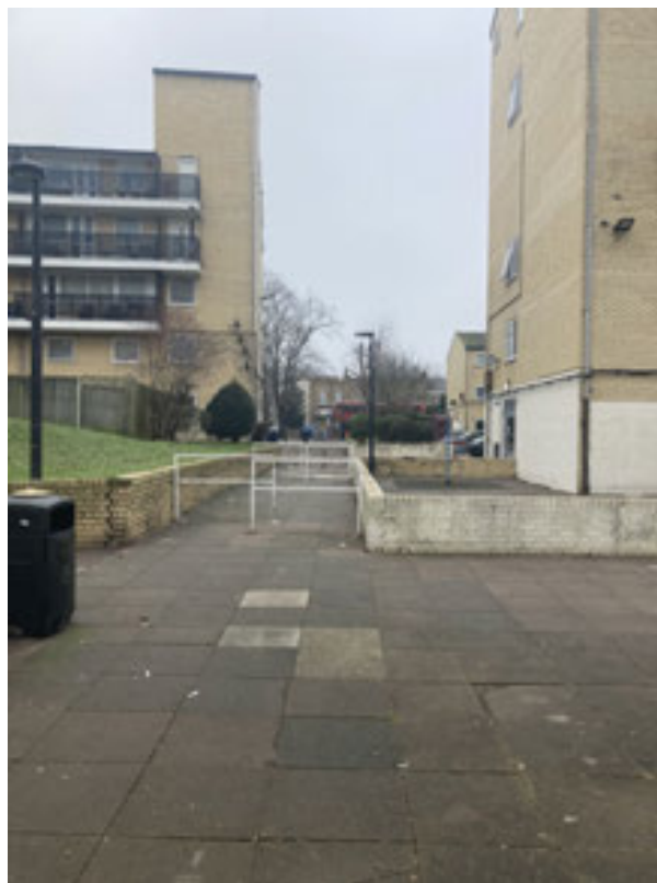
Plate 58: Further west alongside Wilmot Close and looking towards Peckham Hill Street some changes in levels is evident here, but relate solely to the layout of the estate in the 1950s and are not archaeologically significant.
