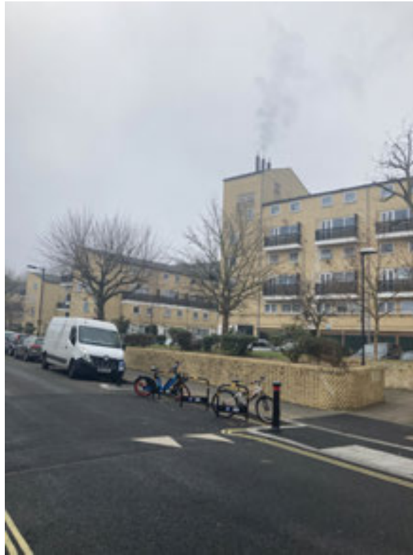
Plate 53: Route of DHN pipes south down Furley Road, to join the Boiler House at the Bells Gardens Estate
