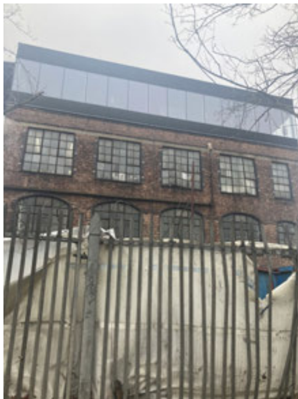
Plate 6: Warehouses surviving on the southern side of the Grand Surrey Canal on Surrey Canal Road, a reminder of the industrial heritage of the area.
