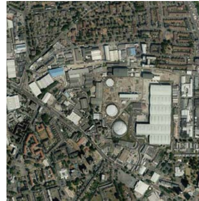
Southwark integrated waste management facility
