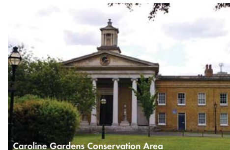
Caroline Gardens Conservation Area
