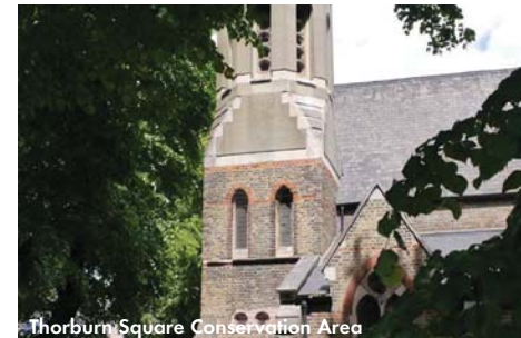
Thorburn Square Conservation Area
