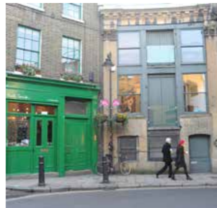
Shops and converted warehouses, Park Street
