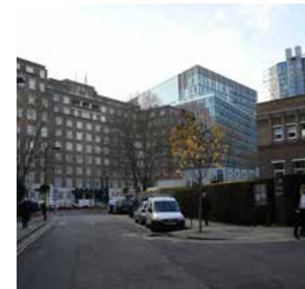
Tall buildings including Bankside Mix
