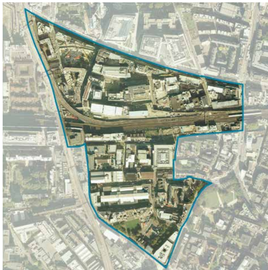
Figure 45: Bankside Commercial - Aerial Overview
