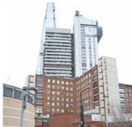
Tall building cluster at Guy's Hospital
