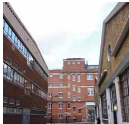
London Fire Brigade Buildings, Copperfield St.
