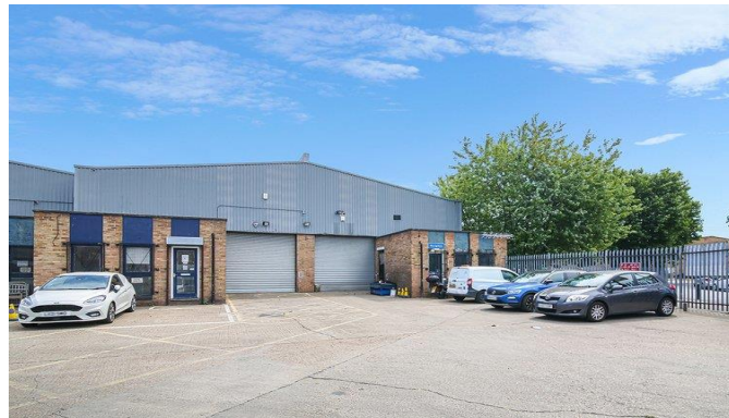
Sandgate Industrial Estate (Site 5)
