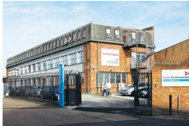
53 Sandgate Street (Site 1)
